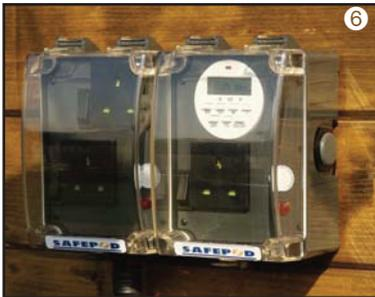
The second module must also be secured to a rigid surface (6). A third module can be added in a similar manner. Ensure that the power consumption does not exceed 10 amps.
